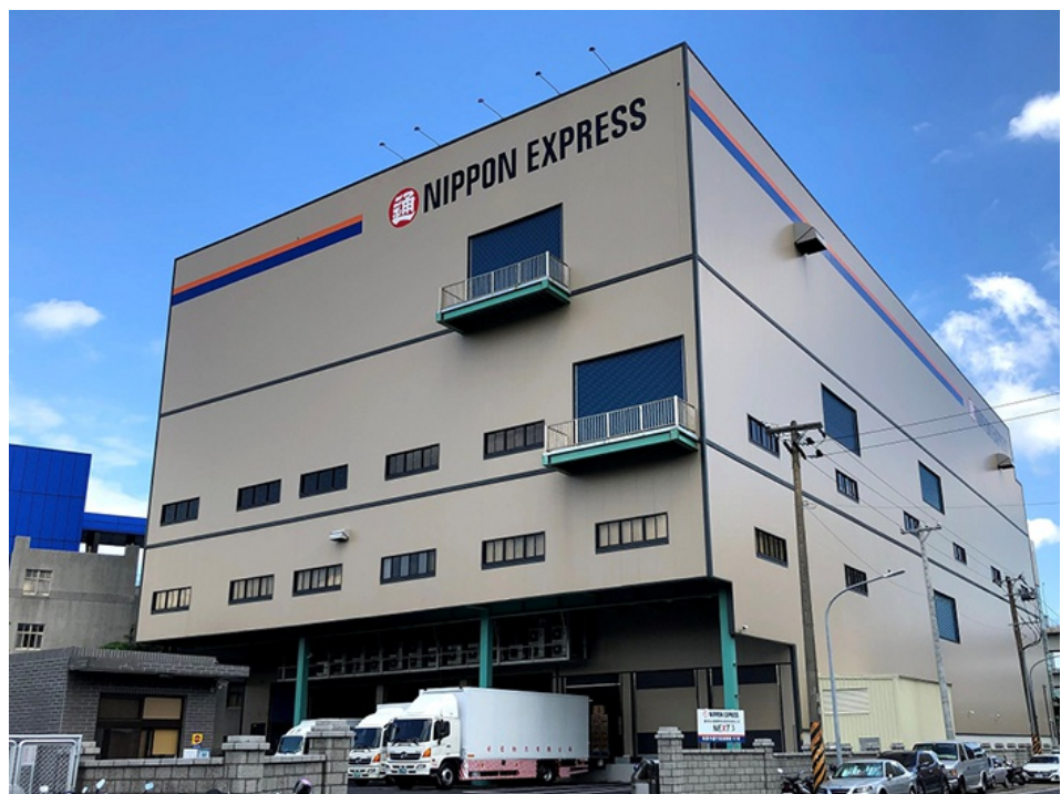
(NEXT3倉庫外観)
